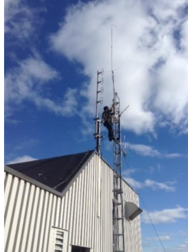
Raising the antenna
